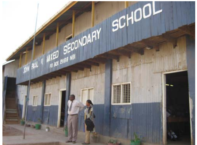
Main building of John Paul II Mixed Secondary School in Kibera, recently painted with the funding from Rockbrook School of Ireland
