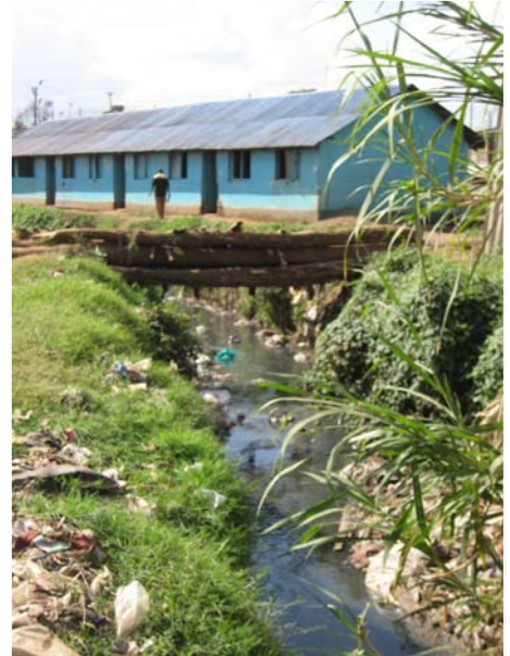
Background: Main building at St. Gabriel Academy. Foreground: Old access bridge over sewage trench
